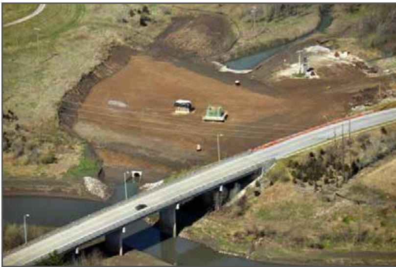
Blue River Basin Levee Improvements
