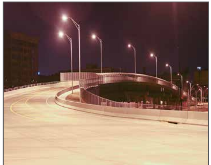
Completion of the Forrester Viaduct
